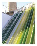
Figure 4 Smokestack emissions bubble through algae-filled tubes at MIT's Cogen plant. (Photo: Ashley Ahearn)
