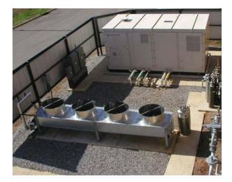
Figure 8 Fuel cell installations at ORNL
